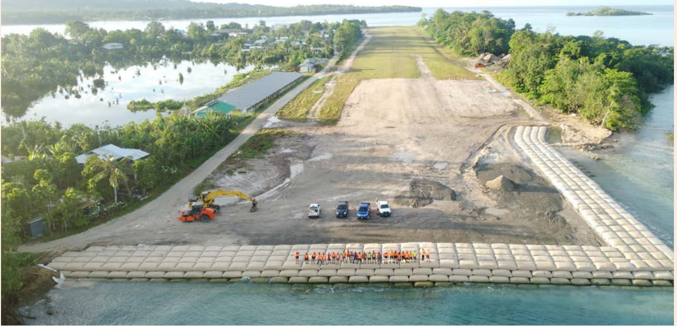
Taro Island, Choiseul Airport seawall construction as part of Solomon Islands Provincial Airfields Upgrade. The team shown is primarily local workers who are engaged and trained by Downers as part of the Ministry's commitment to leave a legacy behind in trained staff, and to provide local employment. 80% of all staff on this project are locally resourced. Credit: Downer Group.
