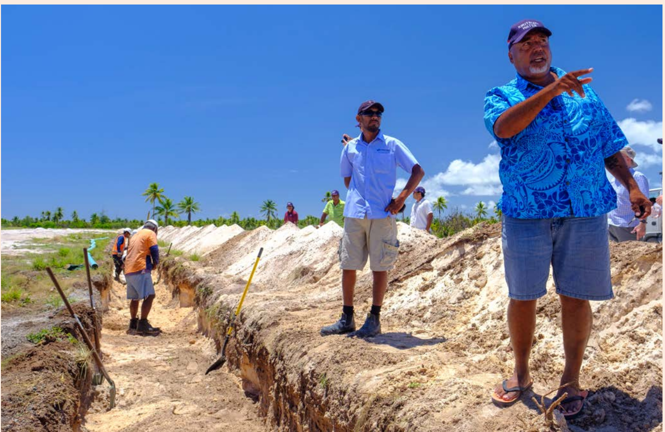
Kiritimati Island Safe and Secure Drinking Water project. Credit: SPC
