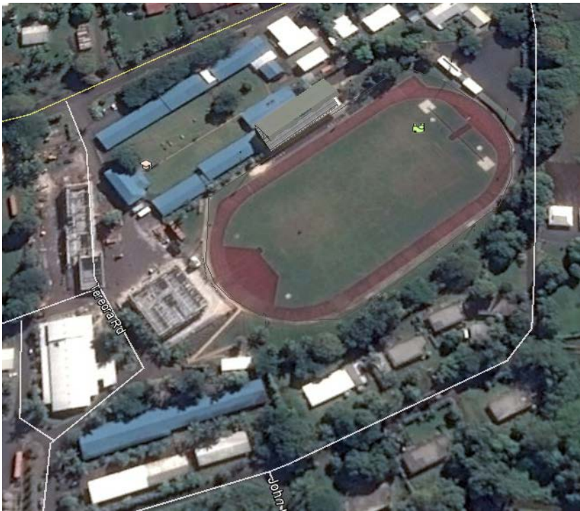
Figure 1: Tereora College site, showing foundations of Stage 1 buildings under construction (Source: Google Earth)
