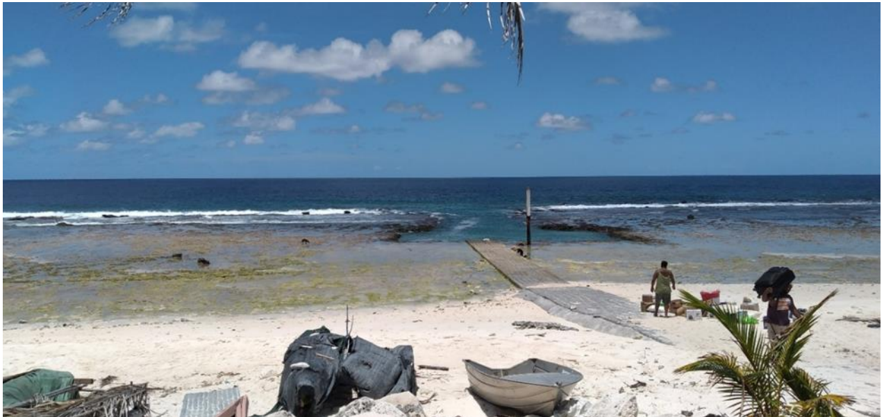
Figure 6: Legacy Ship to Shore Infrastructure on Niutao
